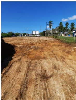
The East-West Arterial Project Photo Courtesy: NRA
