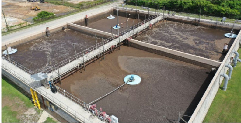
The motor for the ASD was replaced at the Wastewater Treatment Plant
