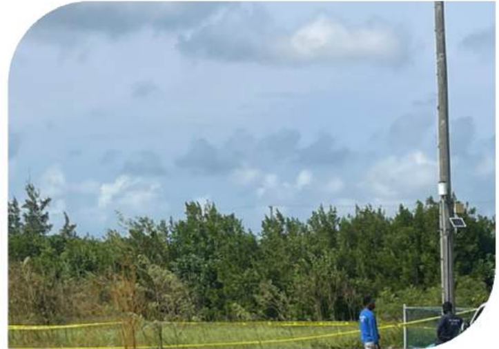
Installation of IoT Flood Sensor in Bodden Town, Grand Cayman.
