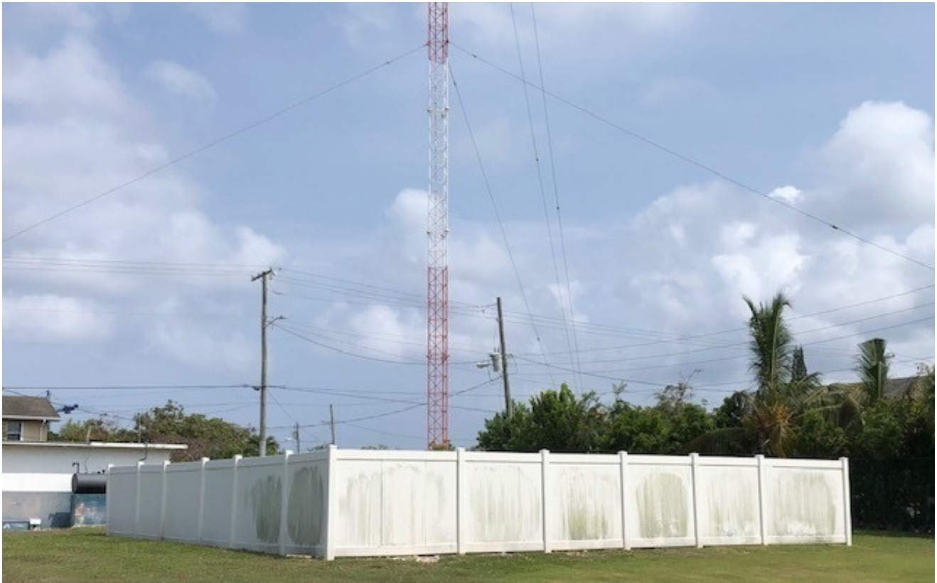
The 120-foot-high Non-Directional Beacon off Walkers Road, once used to navigate aircraft to Owen Roberts International Airport, was dismantled.
