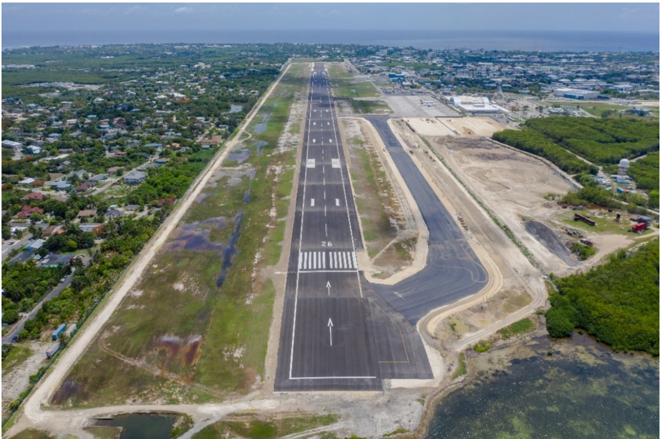
ORIA Airfield Upgrade Project underway, June 2020
