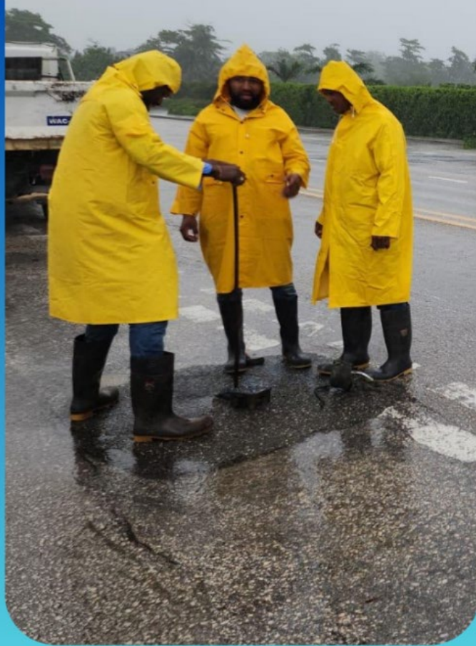
Water Authority crews restoring water service following Hurricane Beryl.
