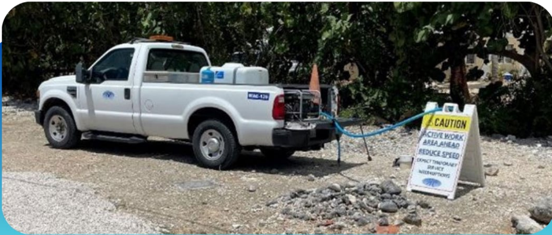
Water Authority conducting leak detection work in Cayman Brac.
