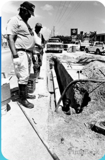
Water Authority staff installing pipeline is one of many photos featured in the TimeBack project. Photo Courtesy: Compass Media
