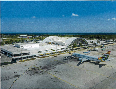
Airside views of the nearly completed new ORIA terminal
