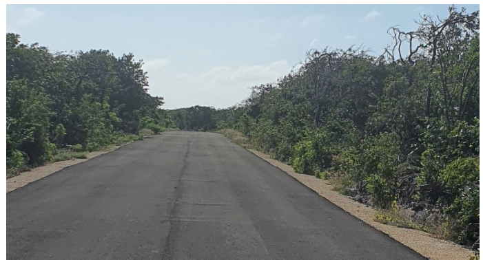
Paved section of "Lemmie's Farm Road".
