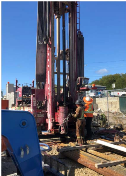
Drilling of test wells for hydrogeological study to use groundwater for cooling of the Energy Recovery Facility.
