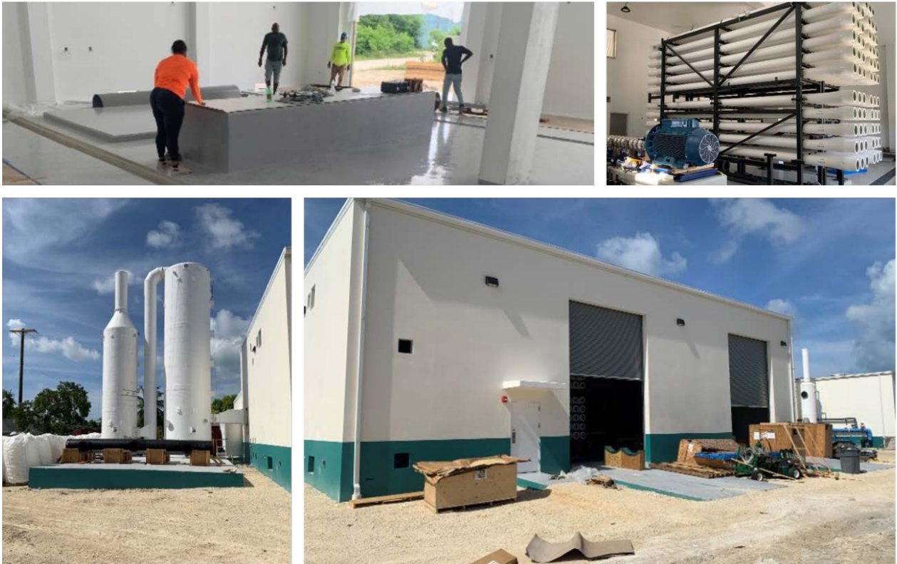
Construction process of the new RO Plant.
