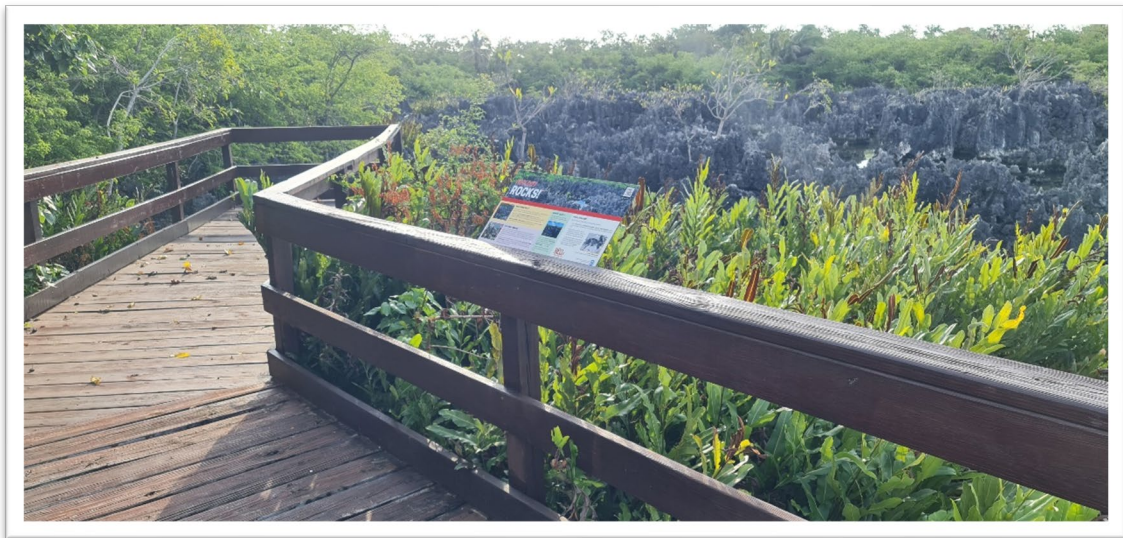
Figure 43: Additional signage installed along the boardwalk.
