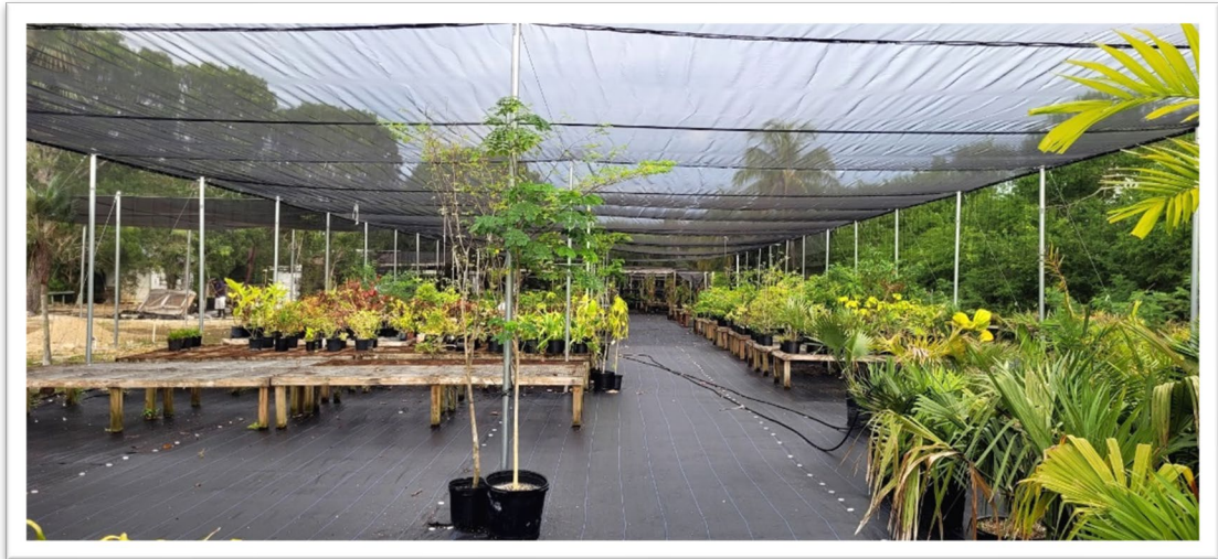
Figure 25: Nursery renovations nearing completion.
