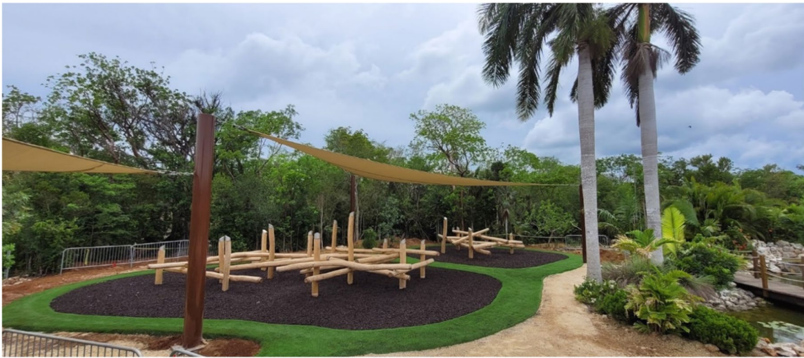
Figure 32: Final pathway works and placement of safe fall material for the Children's Garden climbing structure.
