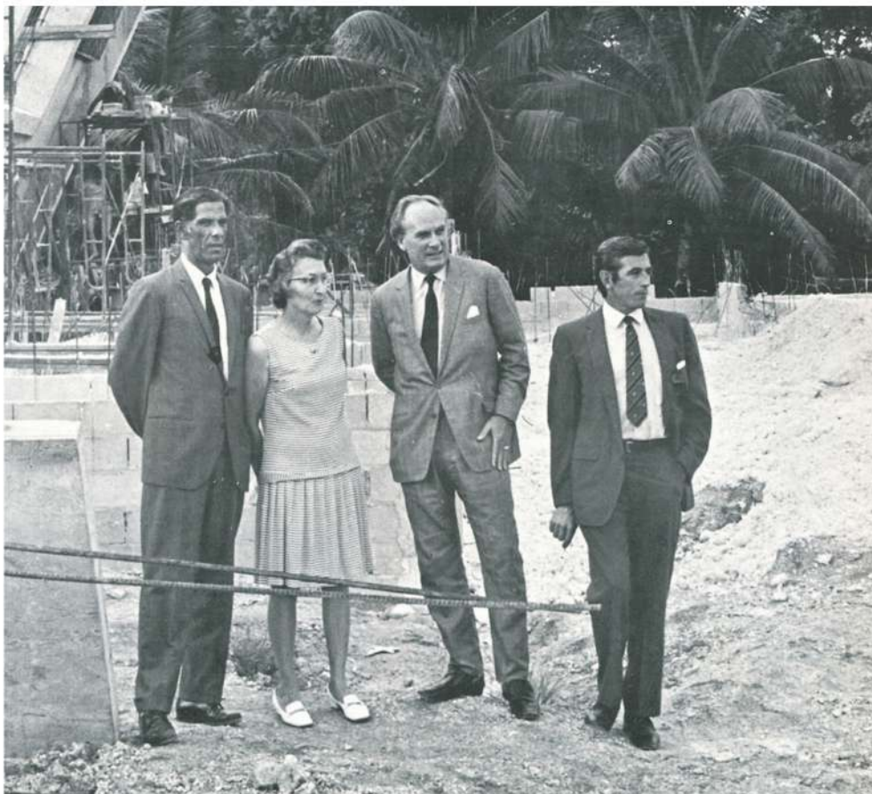
Left: (Left to Right): Deputy Governor Mr. Desmond Watler, Mrs. Watler, Governor A. Long, and Resident Architect Jack O'Connor inspecting the construction of the Legislative Assembly Building, September 1971. (Compass Media Ltd.)
