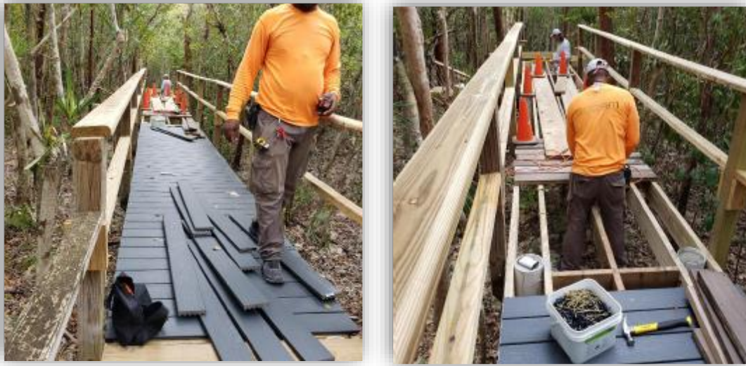
Figure 15 - Workers reconstructing the Orchid Boardwalk
