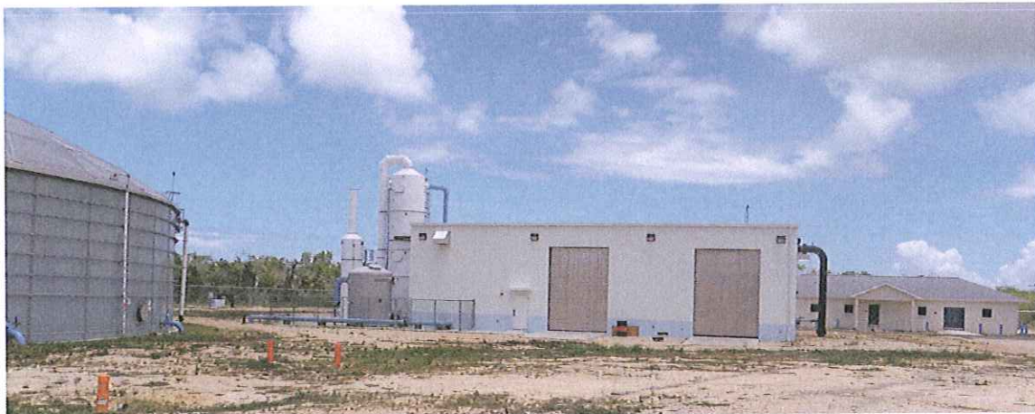
North Side Water Works - June 2009
