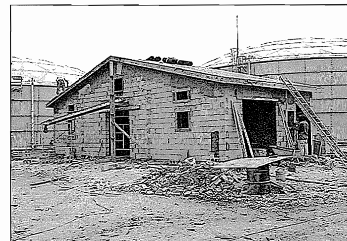
Construction on the Lower Valley Pipe Storage and Workshop Facility
