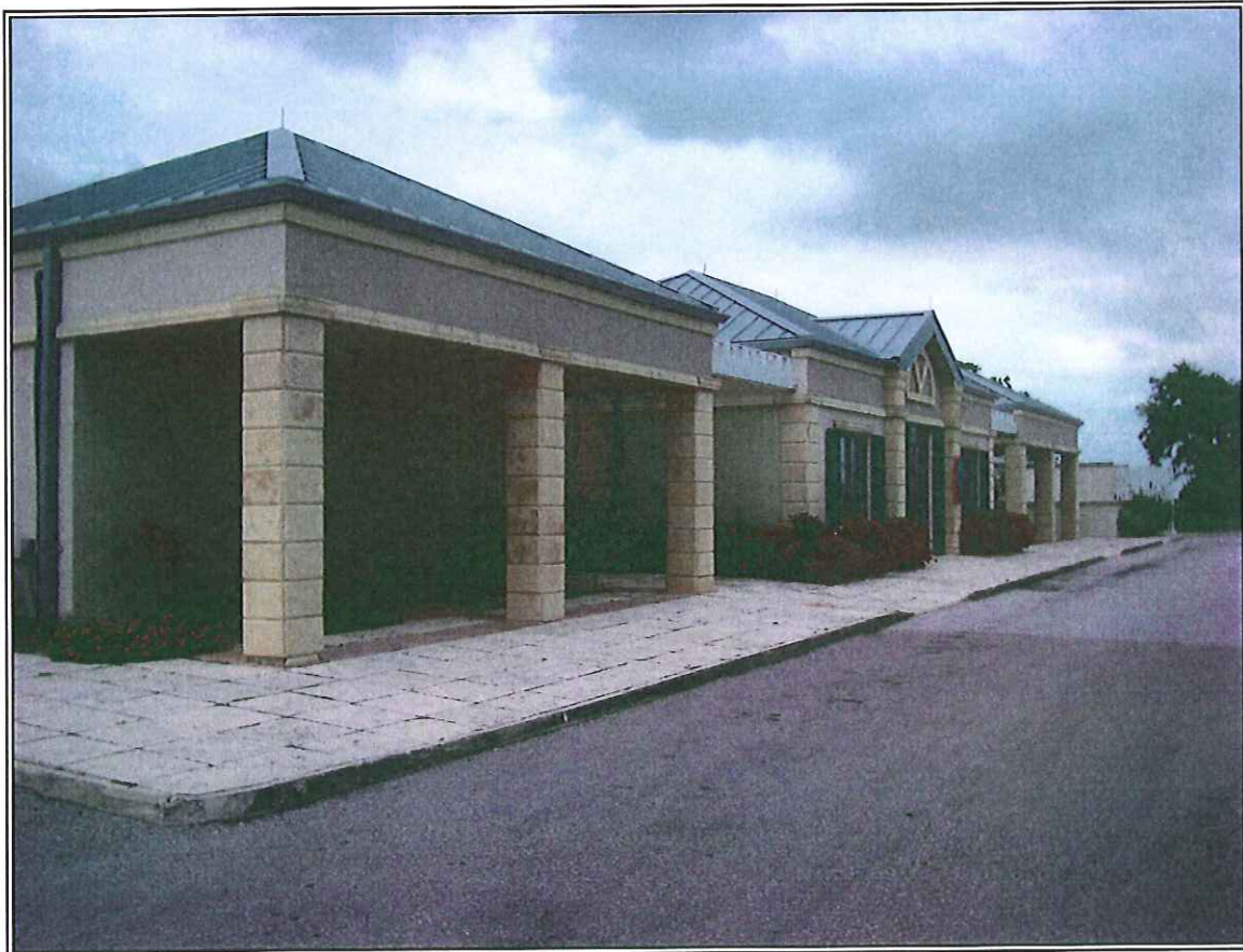
Visitor Centre (from car park)
