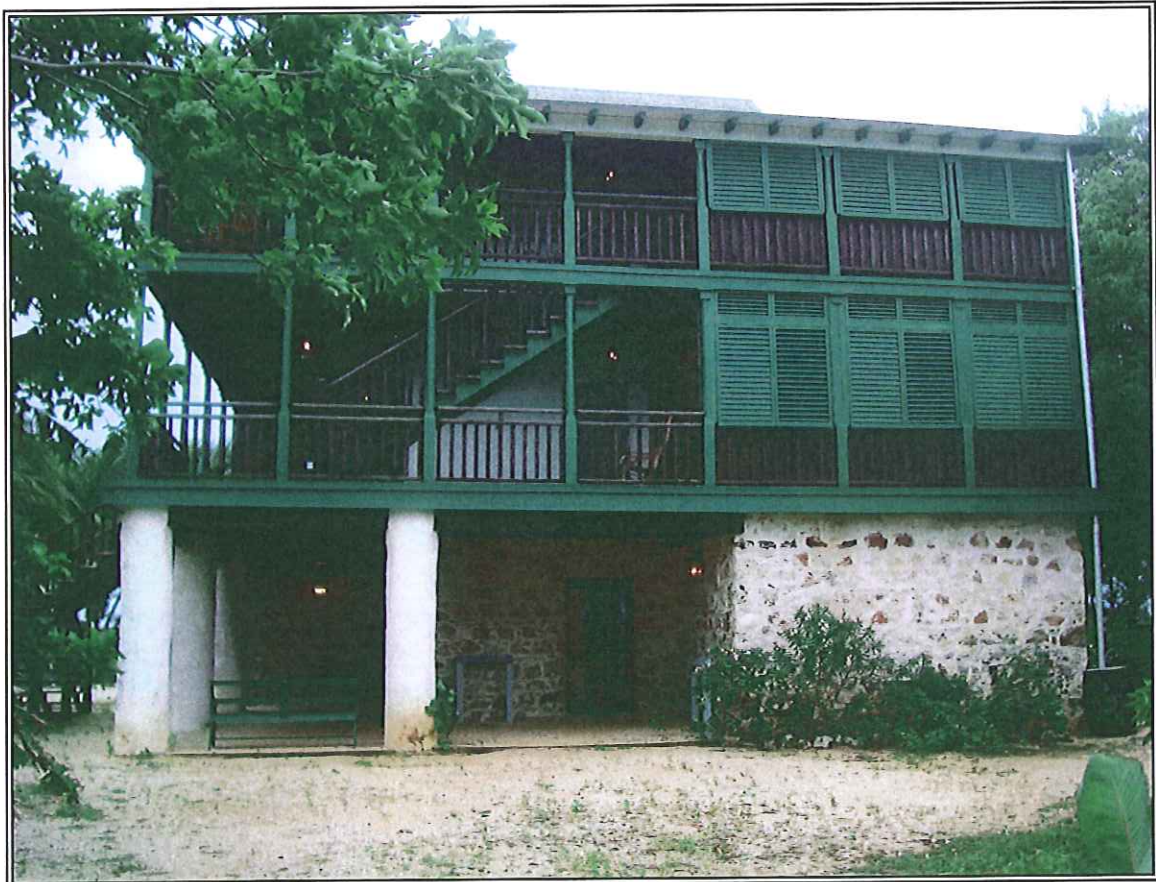
The Great House (northern elevation)
