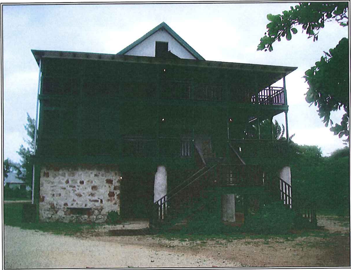
The Great House (eastern elevation)
