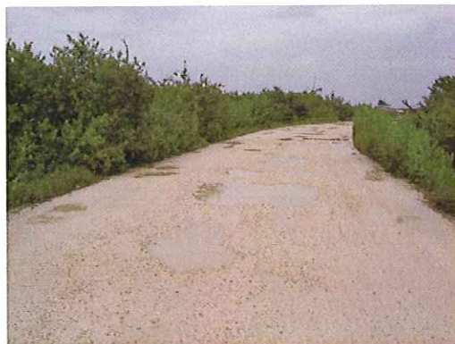
ROUGH GRADED ACCESS ROAD – LAKE DESTINY DRIVE
