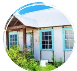
December Nixon House Relocation Project underway
