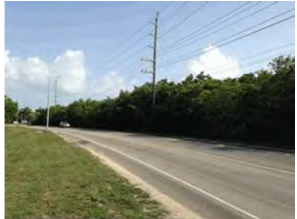
Photo# 2 Facing South Along Esterly Tibbetts Highway
