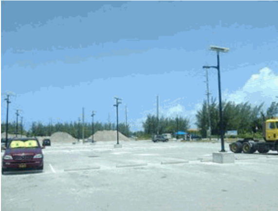
View of Portion C Looking East
