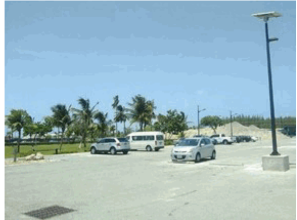
View of Portion C Looking East
