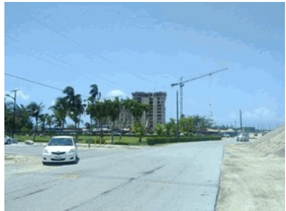
View North along Interior Dividing Road
