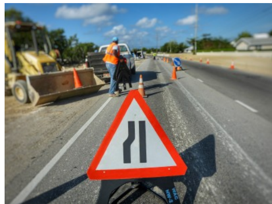
ClickB4UDig is an industry initiative protecting the safety of workers and underground infrastructure throughout the Cayman Islands (photos from WAC)
