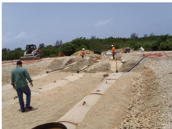
OfReg inspectors at site for the installation of new underground fuel tanks
