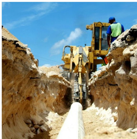
Installation of a potable water distribution pipeline in the Cayman Islands (photo from WAC)
