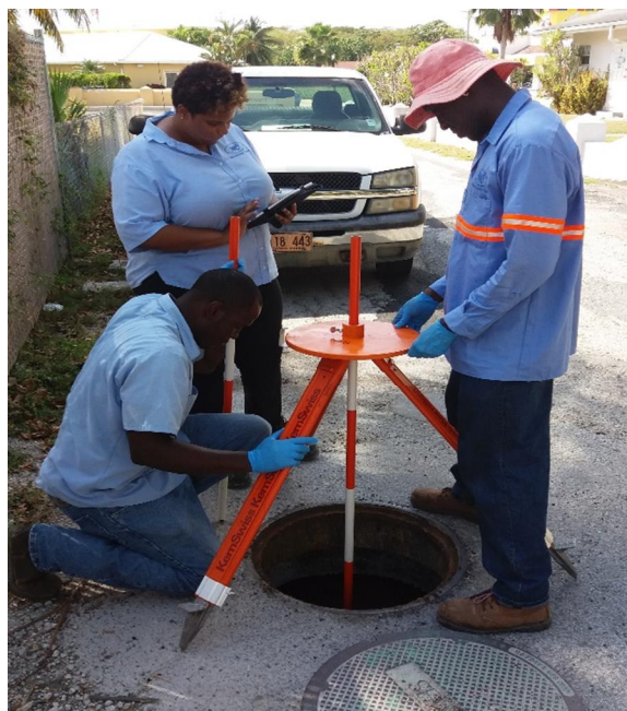
Members of the Wastewater team use a GoPro mounted to a specialty rig designed in-house to survey manholes safely and efficiently.
