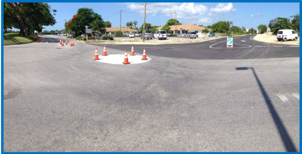
New Mini Roundabout by Owen Roberts Airport
