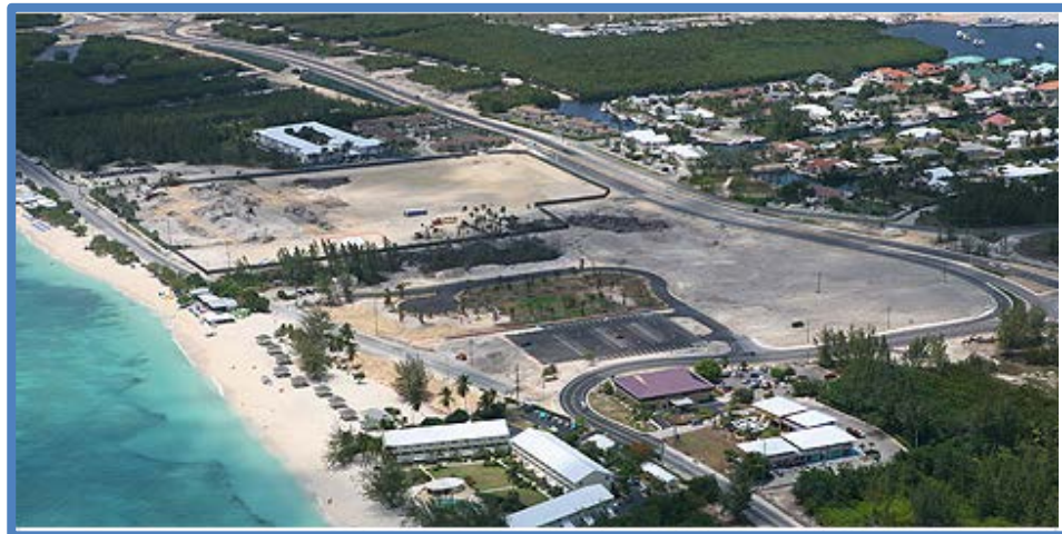
Aerial view of West Bay Road diversion onto ETH at the Public Beach
