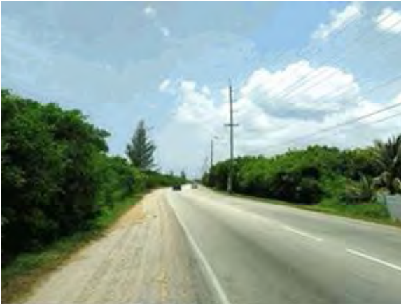
View West Along Highway Block 20D Parcel 175
