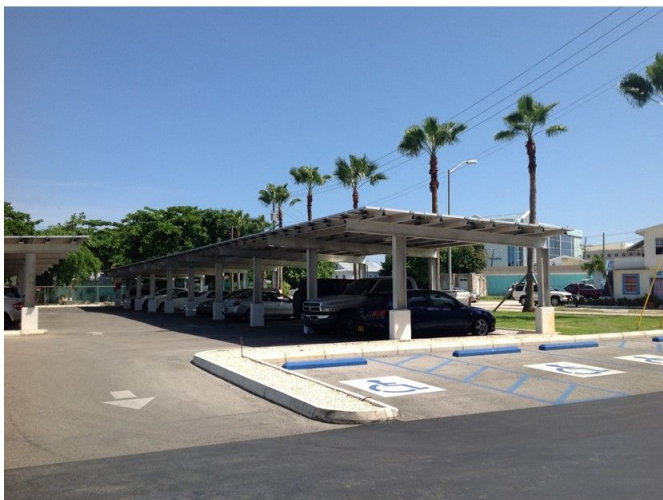
Photo: Engineered car park utilizing solar photovoltaic panels to export energy into CUC's T&D System.
